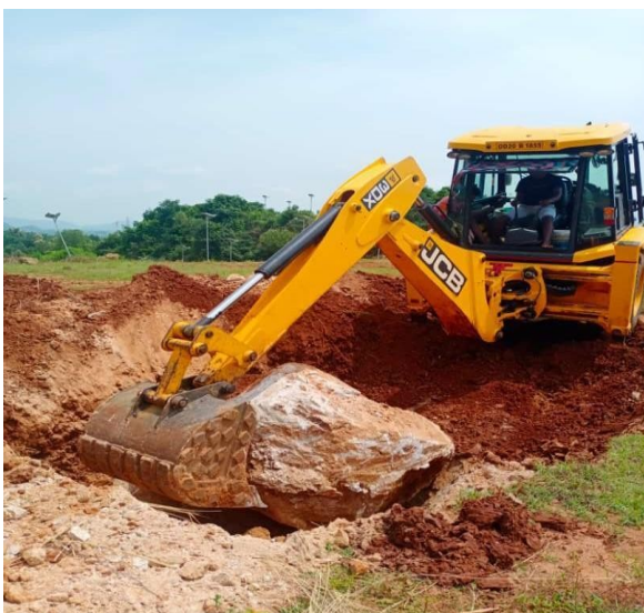
Fig 10: Removal of Boulders
