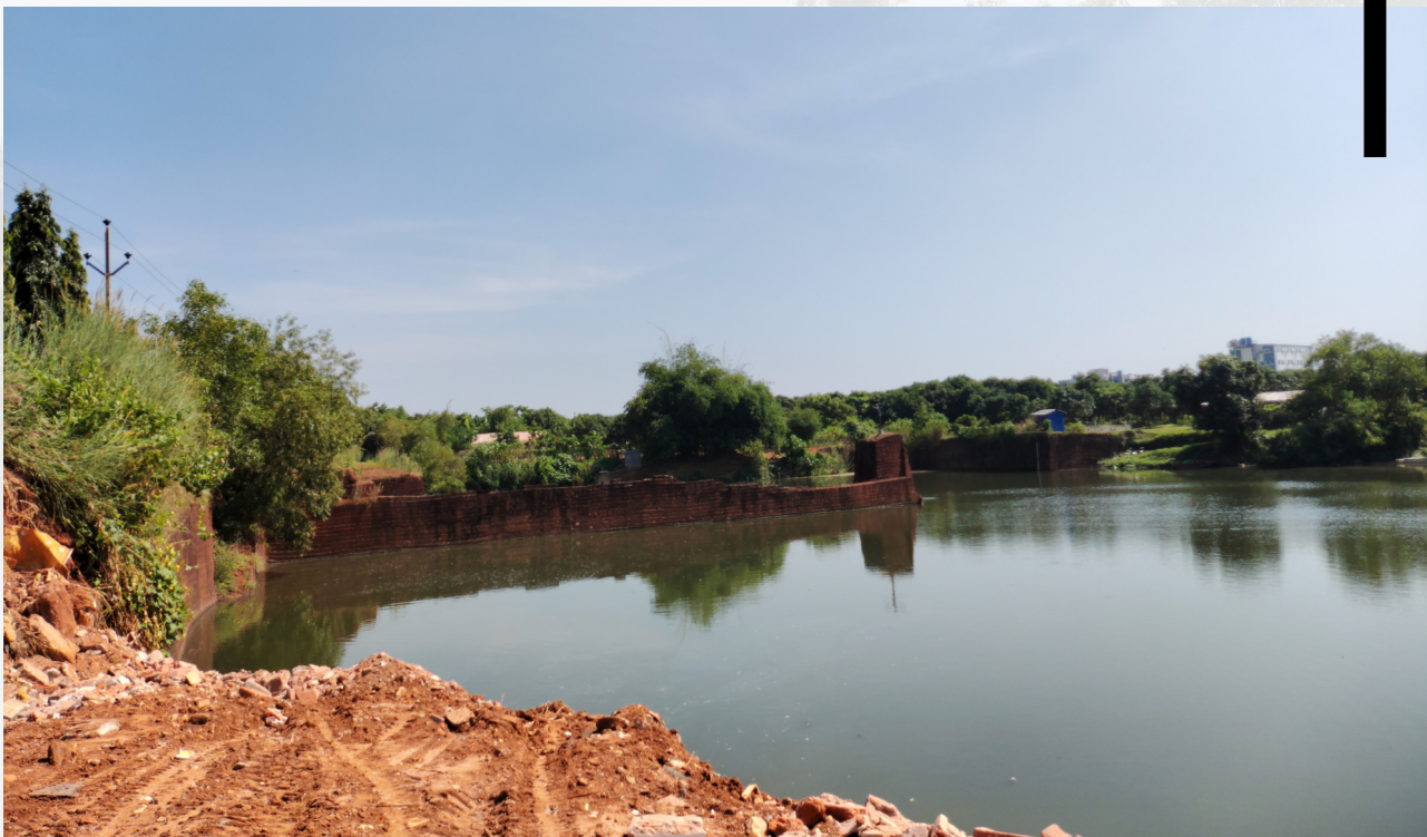
Pits made by illegal mining activity which is transformed for waste water treatment and RWH
