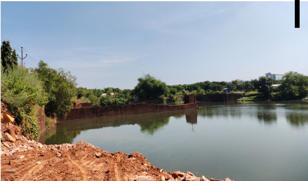
Pits made by illegal mining activity which is transformed for waste water treatment and RWH
