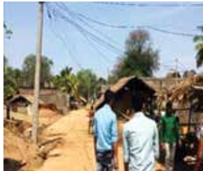
Construction of Pakka Roads
