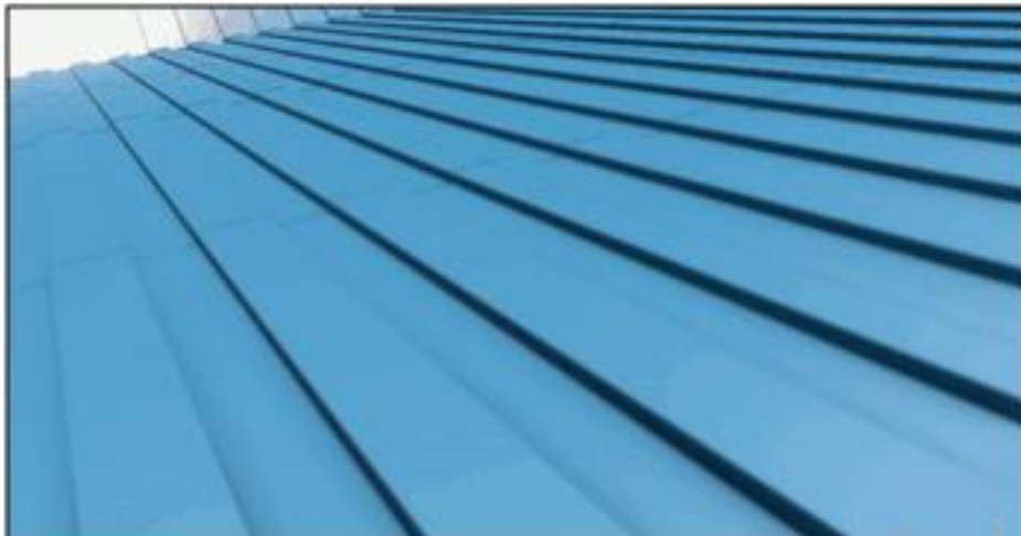
Walk Through of Foot Over Bridge
