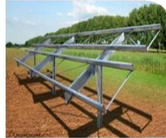
Module mounting structure is used to fix solar panels on surfaces like roofs or the ground
