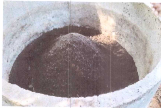
Installed Cement Ring
