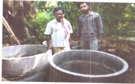
Installed Cement Ring
