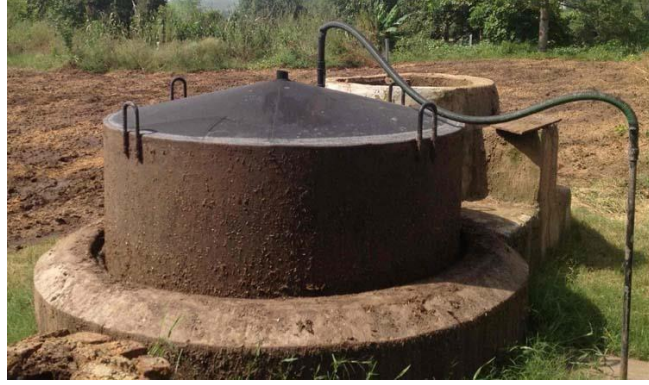
Fig: Food waste and cow dung digester (Biogas plant) for generation Biogas in tribal village, CUTM
