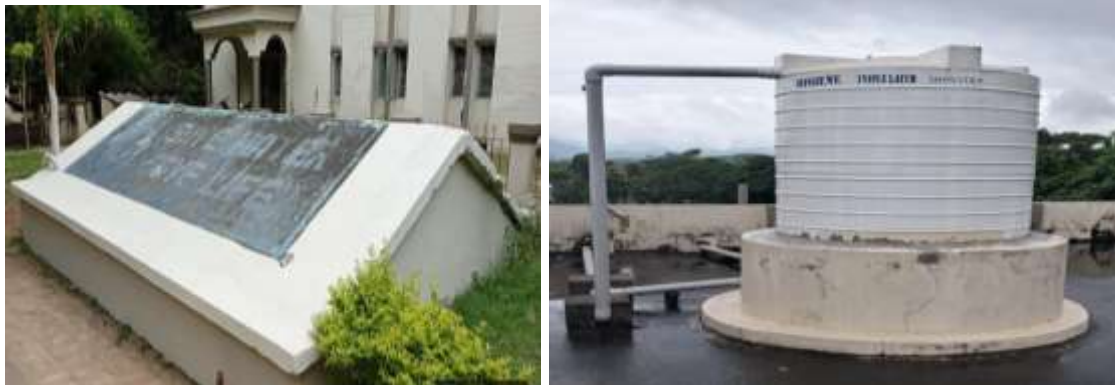
Figure: 1.4- Image of Overhead Tank and Sump
