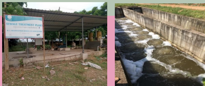
Sewage Treatment Plant (STP)
