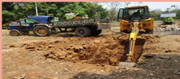
Excavation of land for Chinese Circular hatchery
