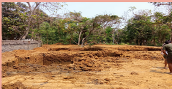
Excavation of land for AS
